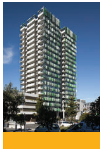
P.67 Off-white Burlesque Bricks complement over-scaled black window boxes. P.69 A high performance facade includes external perforated mesh sun shading in a varied colour palette.
